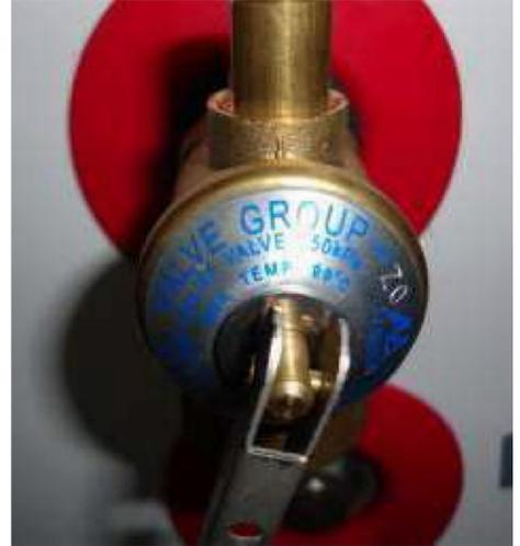
**WARNING** Fail to operate the relief valve easing gear at least once every six months may result in the water heater exploding. Continuous leakage of water from the valve may indicate a problem with the water heater.
